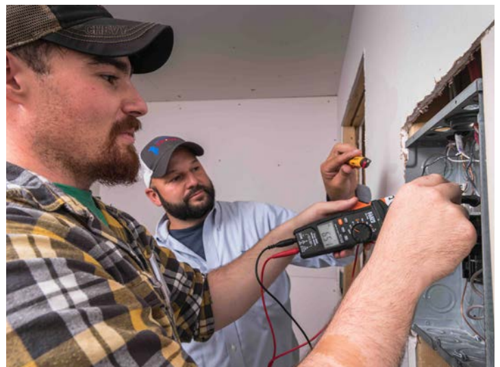
Student working with instructor on troubleshooting electrical issues in the breaker panel.
