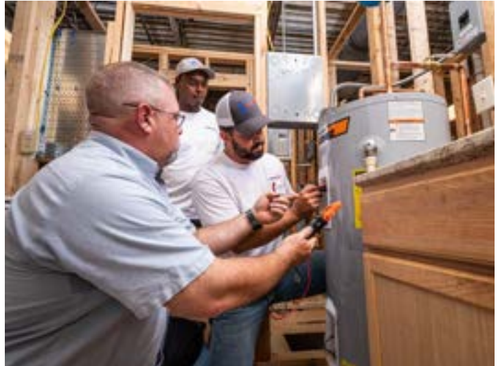
Plumbing students troubleshooting on an installed hot water tank.
