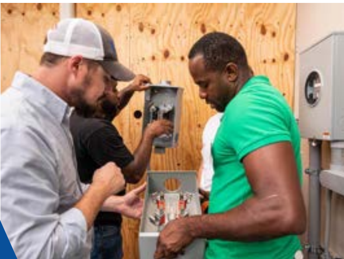
Students setting breaker panels and breakers into boxes.
