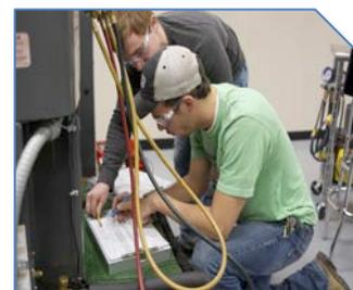
Students fill out Total Tech's Troubleshooting Guide to determine which component is giving the heat pump system problems.
